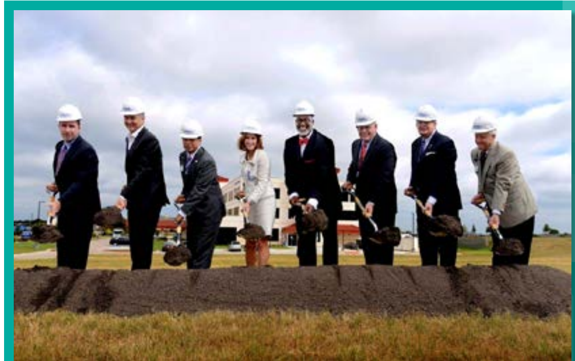
Texas Health leaders break ground on a new medical office building to serve the North Texas community.
